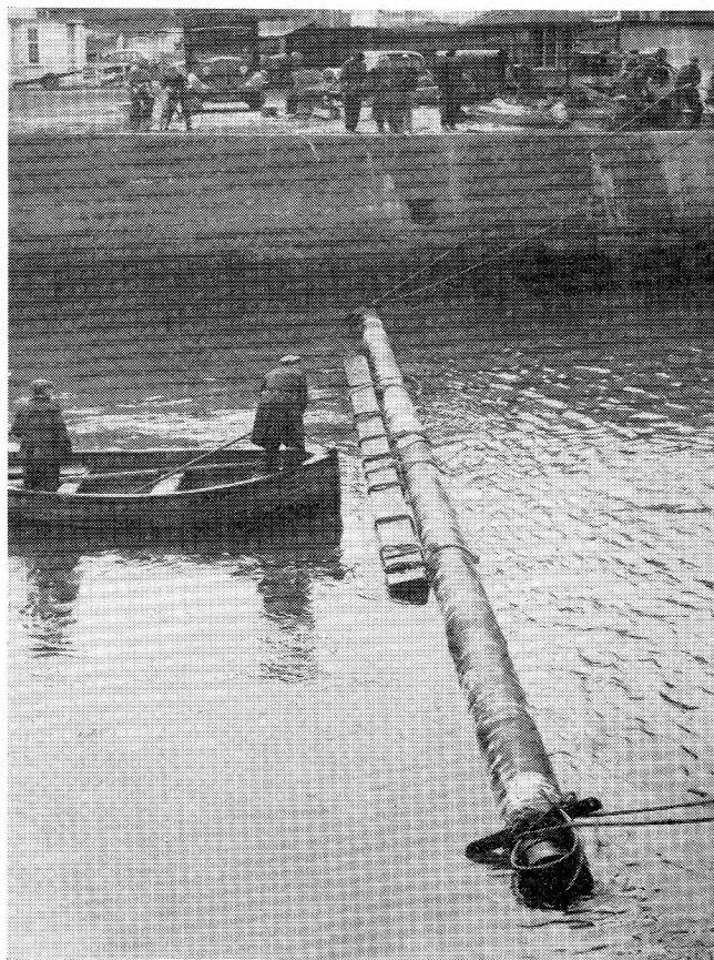
FIG. 10—MAIN-CROSSING PIPE BEING FLOATED INTO POSITION
