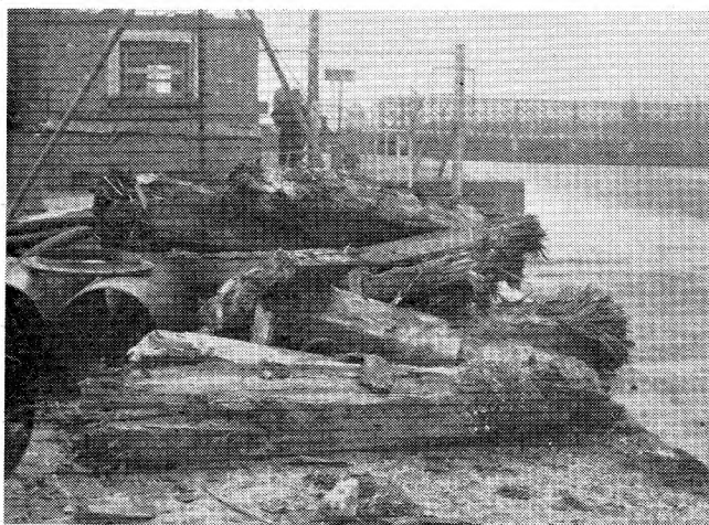
FIG. 8—OLD PILES DREDGED FROM HARBOUR BED
