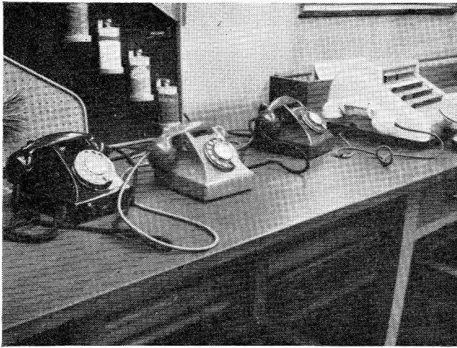
HULL EXHIBITION: SWITCHBOARD AND TELEPHONE INSTRUMENTS
