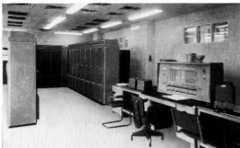
FIG. 1—GENERAL VIEW OF THE FIRST COMPUTER ROOM
