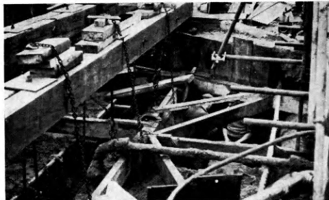
MANHOLE SITE DURING EXCAVATION
