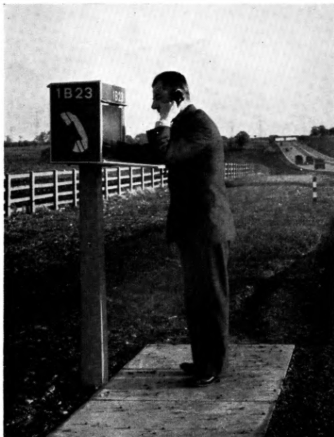
FIG. 4—GENERAL VIEW OF ROADSIDE TELEPHONE
