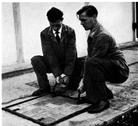
FIG. 8—COMMENCEMENT OF REMOVAL OF MANHOLE COVER
