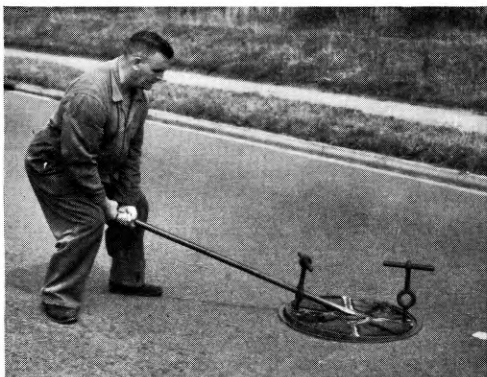
FIG. 7—EASING A MANHOLE COVER USING A CROWBAR
