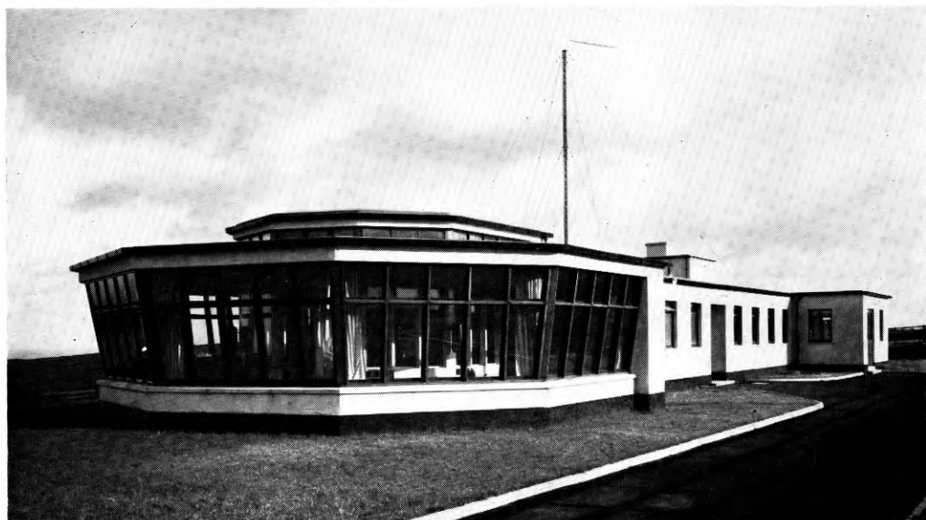
The operations rooms are in the foreground FIG. 1—MAIN STATION BUILDING
