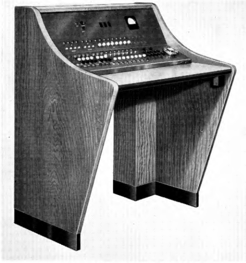
FIG. 4—E.T. NO. 4 CORDLESS SWITCHBOARD
