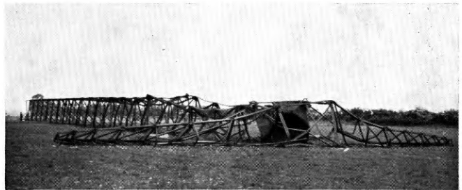
FIG. 2—MAST AFTER BEING FELLED
