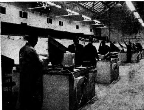
FIG. 5—VIEW OF PRIMARY-SORTING FLOOR
