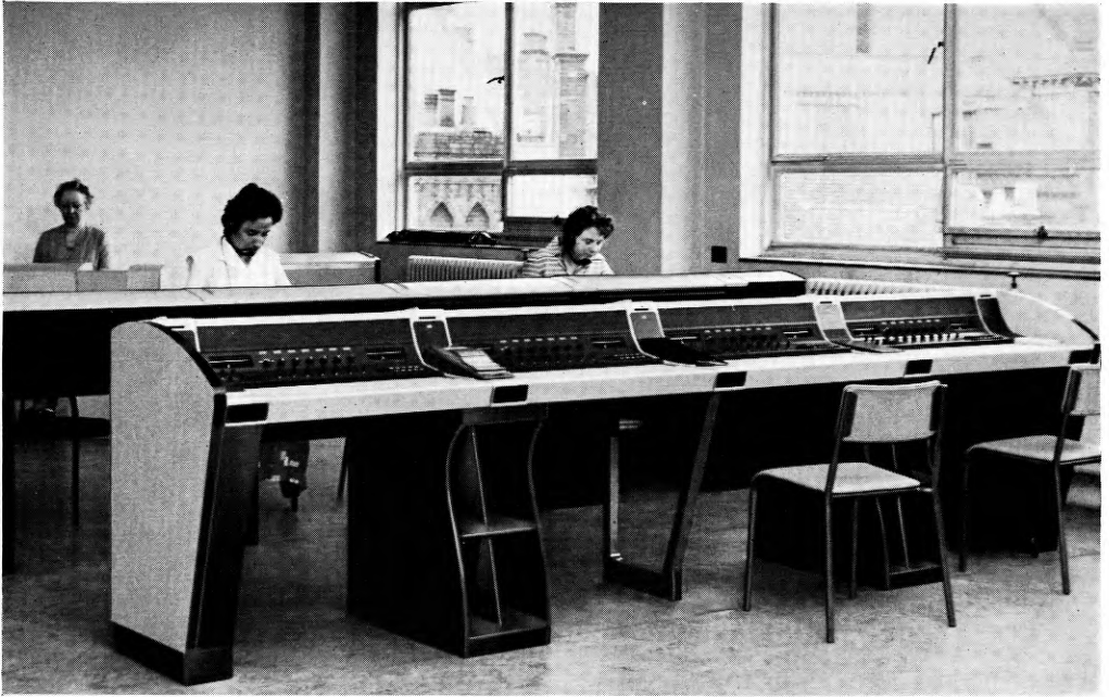
FIG. 2—GENERAL VIEW OF SWITCHROOM
