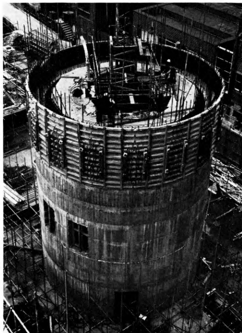
FIG. 3—PROGRESS OF TOWER BY MAY 1962
