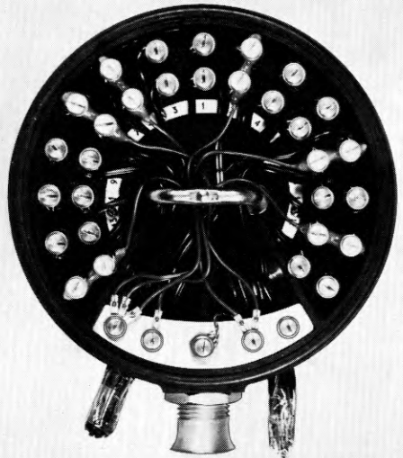
THE MODIFIED BLOCK TERMINAL SHOWING PROTECTORS FITTED TO SIX LINES
