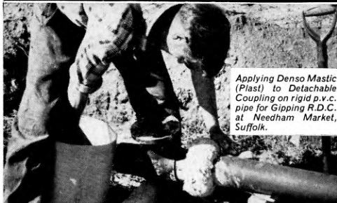
Cable Duct Sealing with Denso Mastic (Plast). Photograph by courtesy of South Western Electricity Board.
