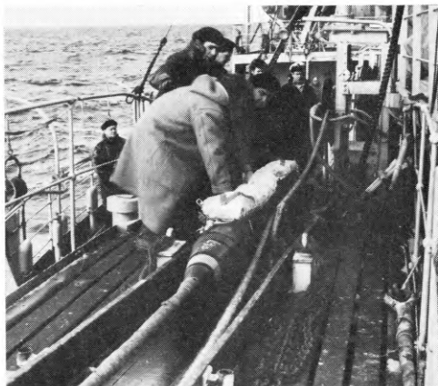
FIG. 5—LAUNCHING A REPEATER WITH PARACHUTE
