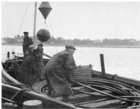
LAYING THE SUBMARINE CABLE TO BROWNSEA ISLAND IN POOLE HARBOUR
