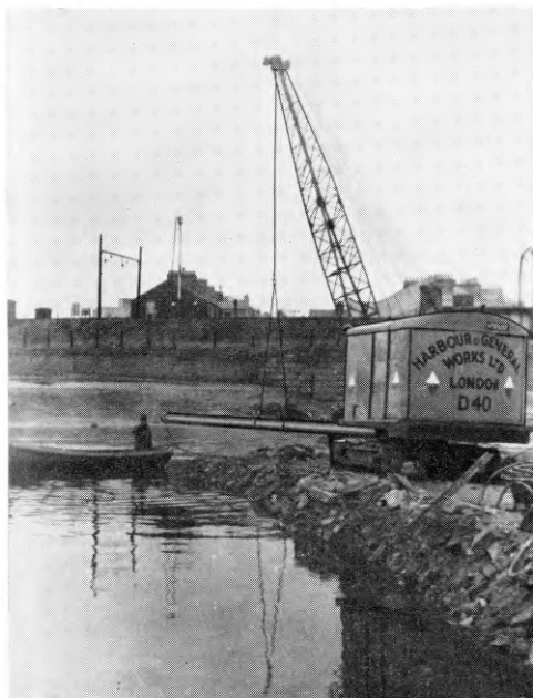
FIG. 2—THE DRAGLINE EXCAVATOR ON THE CAUSEWAY AT THE RIVER LUNE CROSSING
