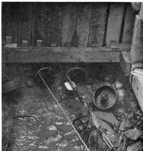
FIG. 6—SWIVELS AND ATTACHMENT PLATE USED TO PREVENT DRAW ROPES TANGLING
