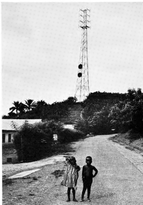
Yagi aerials for a v.h.f. radio-relay system are mounted at the top of the tower; parabolic-dish aerials for a u.h.f. system are fitted lower down FIG. 3—TYPICAL RADIO-RELAY STATION IN NIGERIA
