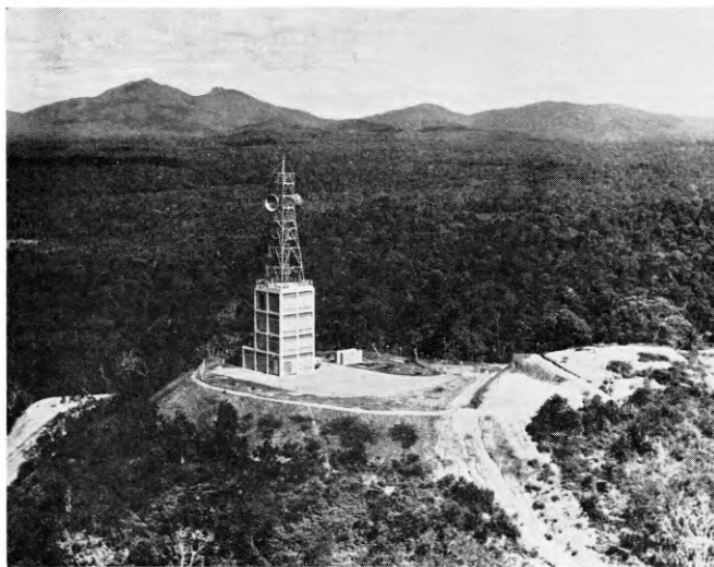
FIG. 5—MICROWAVE REPEATER STATION IN THE MALAYAN KUALA LUMPUR-SINGAPORE NETWORK
