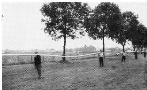
FIG. 5—CONTINUOUS LENGTH OF P.V.C. DUCT
