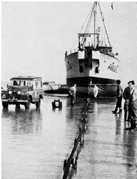
CABLE BEING HAULED ASHORE FROM POOLSTER
