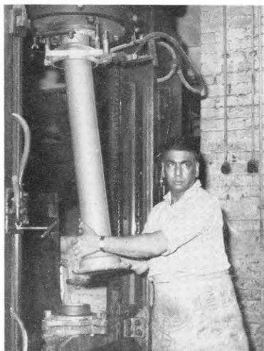
FIG. 4—EXTRUSION OF DUCT
