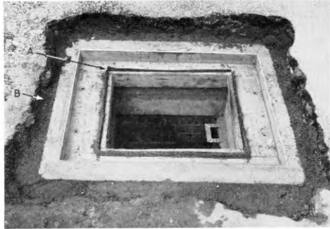
A—Rubber shuttering B—Dry concrete backfill
