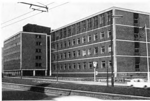
HUDDERSFIELD NEW AUTOMATIC TELEPHONE EXCHANGE
