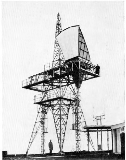
FIG. 8—HORN REFLECTOR AERIAL
