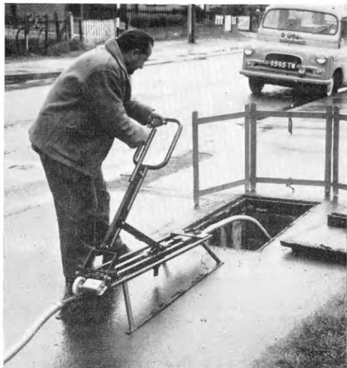
FIG. 3—MACHINE SET UP FOR RODDING A DUCT
