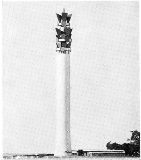
FIG. 11—MODEL OF A MAIN-ROUTE MICROWAVE RADIO-RELAY REPEATER STATION WITH A CONCRETE TOWER
