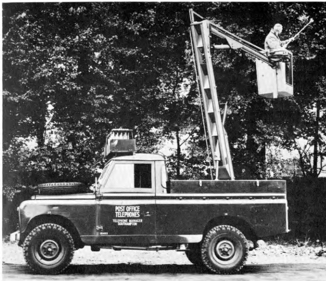
FIG. 2—ELEVATING PLATFORM IN USE
