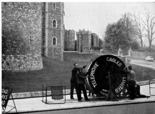
T.C.L. moisture barrier cable at Windsor Castle.
