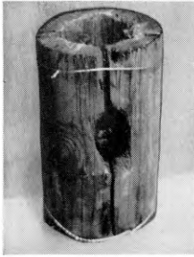
THE SECTION OF POLE DAMAGED BY WOODPECKERS
