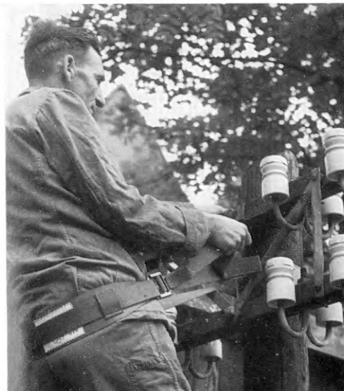
FIG. 3—SHORTENING THE LOOP OF THE POLE BELT
