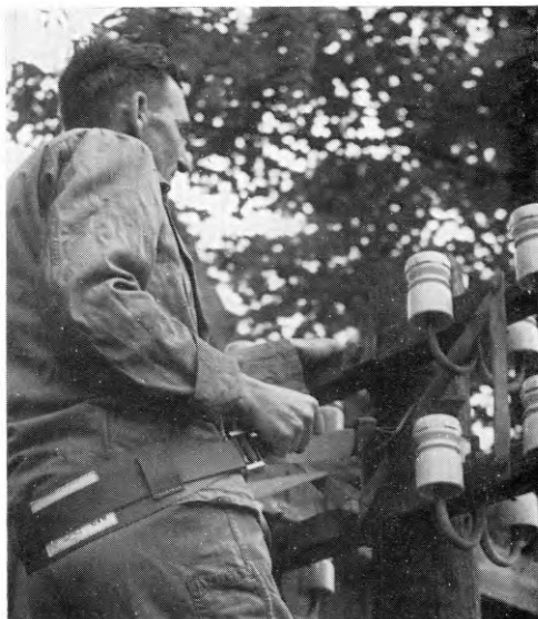
FIG. 4—LENGTHENING THE LOOP OF THE POLE BELT
