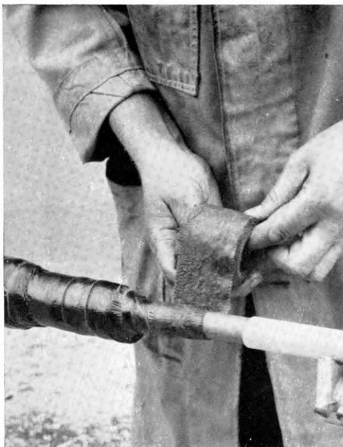
Tape Sealing No. 3 (DENSOPOL ZN) being used to protect a joint in thin lead sheathed, polythene oversheathed cables by the G.P.O. Experimental Jointing Division. Winn & Coales Ltd. have been suppliers to the Post Office of waterproofing and anti-corrosion tapes for over 25 years.
