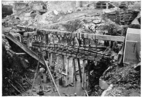
CABLES SUSPENDED OVER ROAD WORKS AT NEWCASTLE
