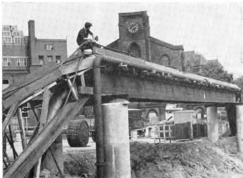
GENERAL CONSTRUCTION OF THE BRIDGE AT CLARENDON ROAD
