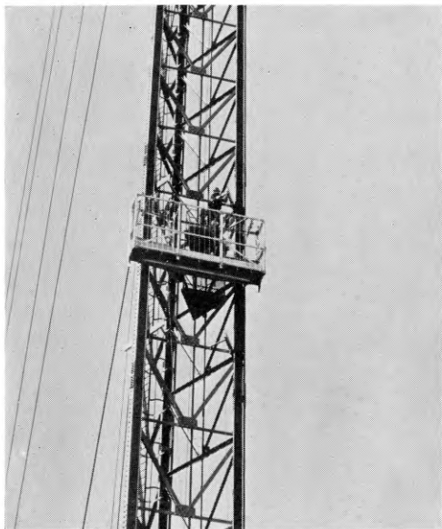
FIG. 9—SKIP IN POSITION ON FACE OF MAST
