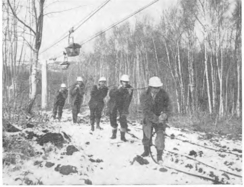
MANHANDLING CABLE BEFORE ERECTION ON THE BUCKET ROPEWAY
