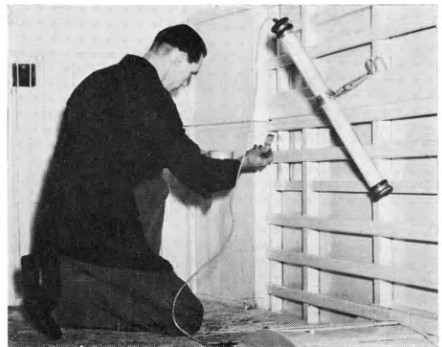
FIG. 8—PORTABLE FLUORESCENT LAMP FOR USE WHEN PAINTING INTERIORS OF VEHICLES
