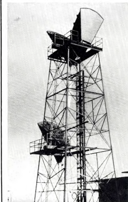
Below: Maxwell's Hill Repeater Station, part of the 6000 Mc/s system in Malaya.
