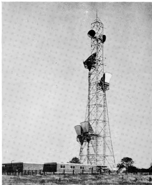
FIG. 6—TYPICAL POST OFFICE MICROWAVE RADIO STATION
