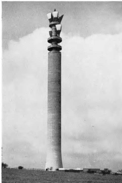
FIG. 3—CHARWELTON RADIO-STATION TOWER
