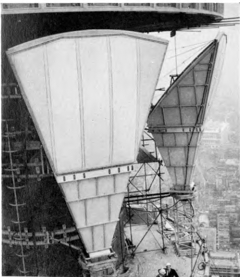
FIG. 10—HORN-REFLECTOR AERIAL BEING INSTALLED ON GALLERY C5
