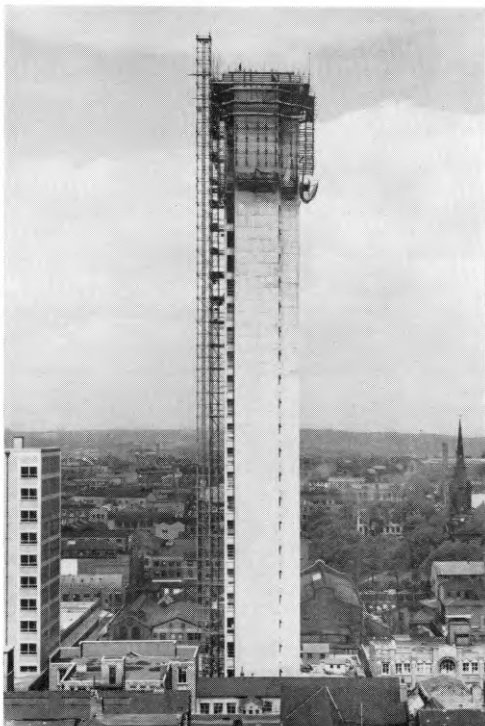
FIG. 3—TOWER UNDER CONSTRUCTION
