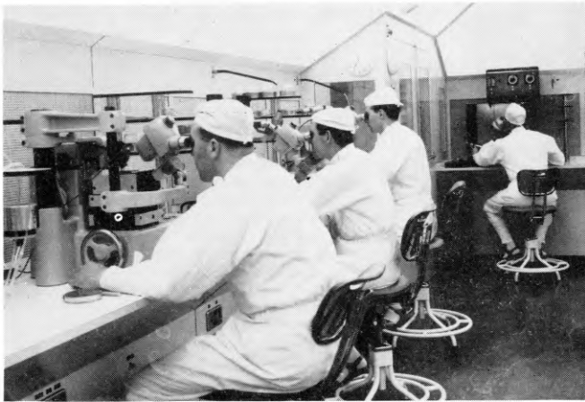
FIG. 5—TWO-PROBE TESTING, DICING, HEADING AND WIRE-BONDING POSITIONS
