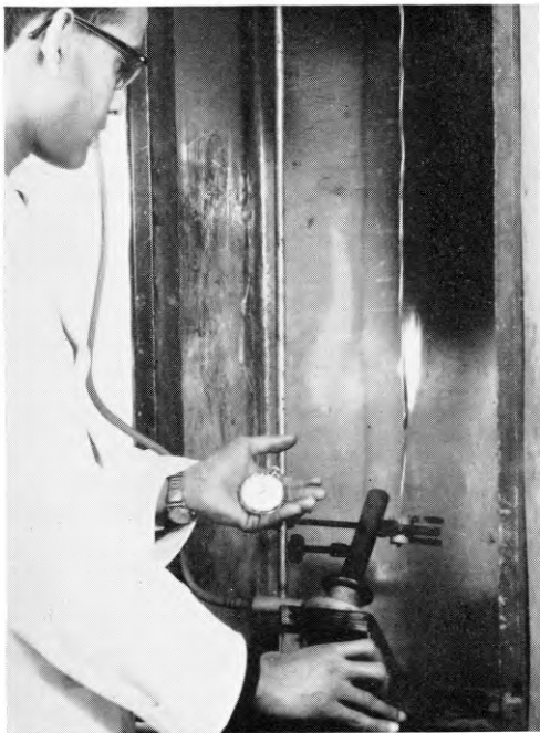
FLAMMABILITY TEST ON JUMPER WIRE
