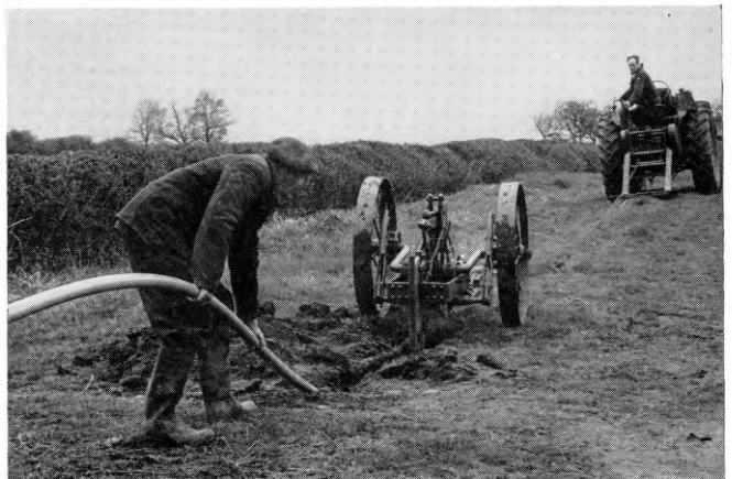
FIG. 7—CONTROLLING ANGLE OF DUCT ENTERING PIT
