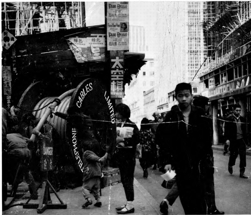
TCL cables being laid in the main business centre of Hong-Kong
