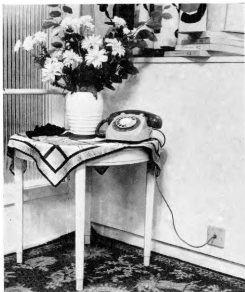
FIG. 2—TELEPHONE TERMINATION INSIDE HOUSE
