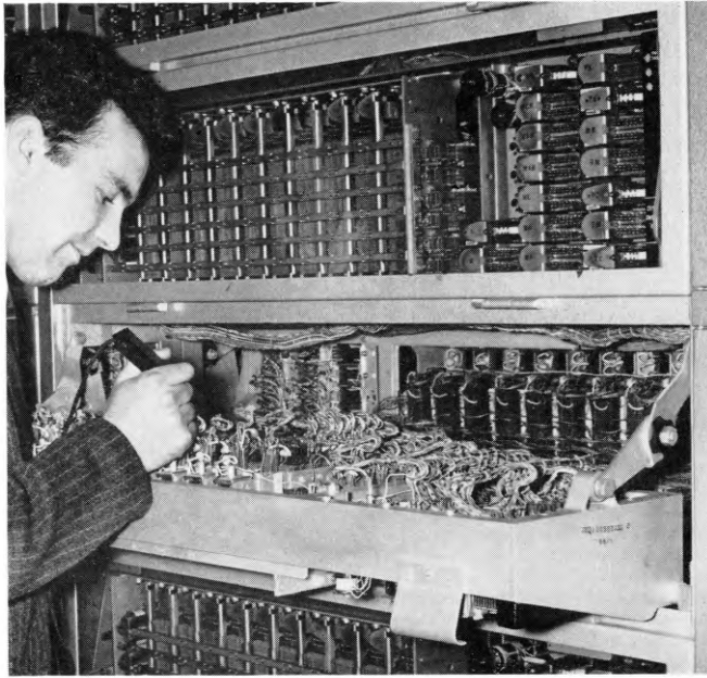
FIG. 12—CHECKING THE WIRING ON A B-DISTRIBUTOR-SWITCH
