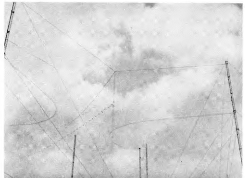
FIG. 11—CONFIGURATION OF THE LOG-PERIODIC AERIAL
