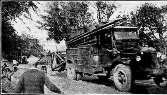
PLACING CABLE IN SHOULDER OF HIGHWAY.
