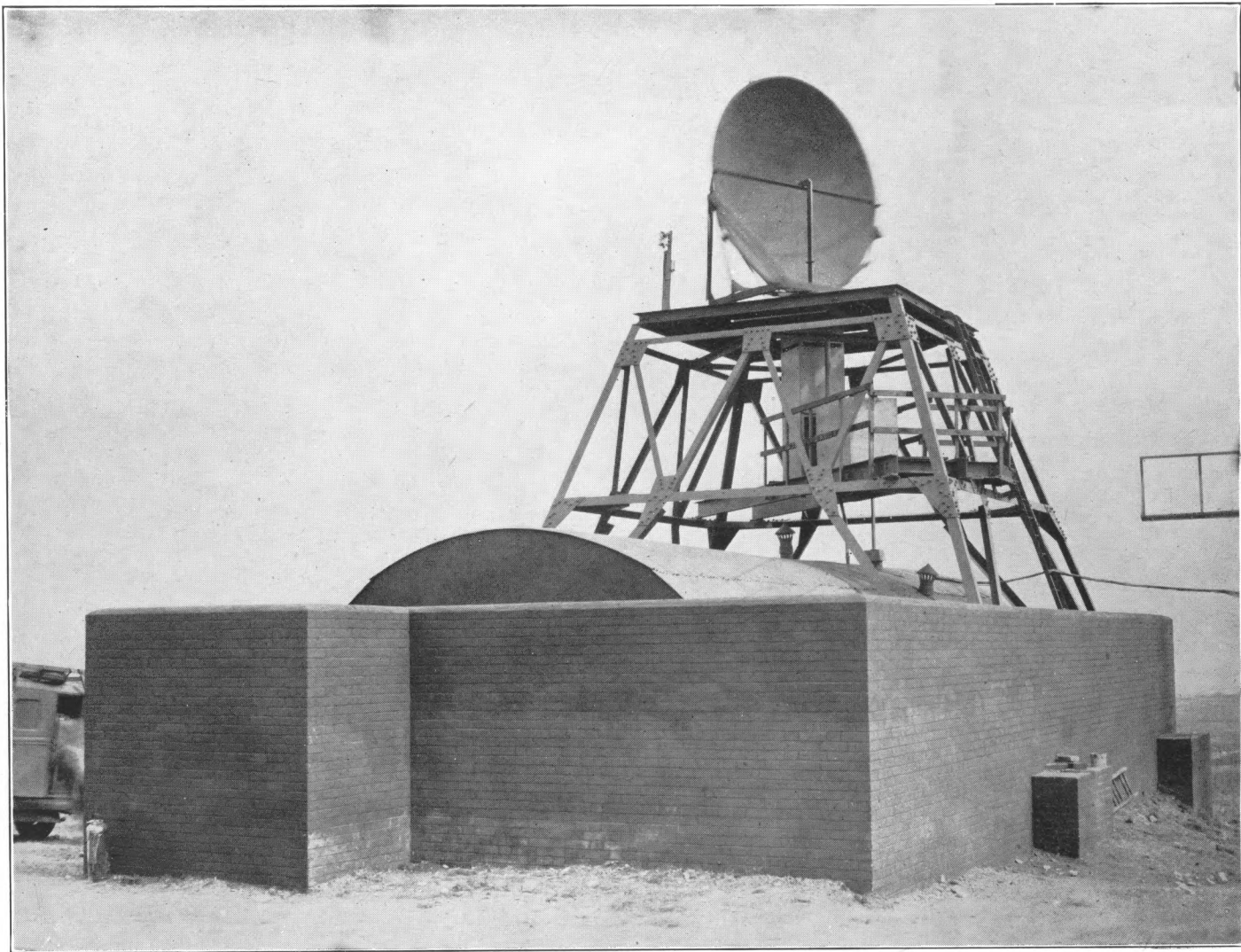
AMES Type 52 with Blast Wall round Operations Hut
