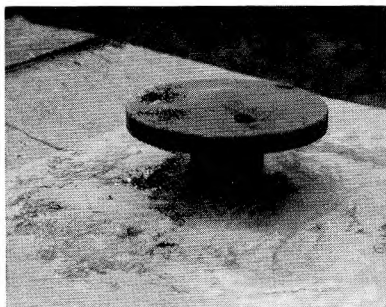
Fig. 4. The base mounting concreted into position
