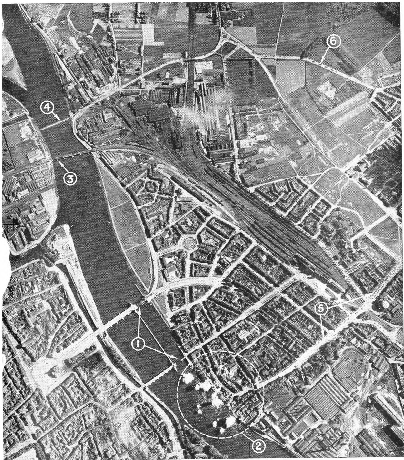
Broken Bridges. A photograph illustrating the great importance of bridge demolition; enemy traffic is delayed and restricted by the work of the Allied sappers at Maastricht. 1, Road bridges under repair. 2, Bombs bursting along the bank of the Meuse. 3, Wrecked span of railway bridge. 4, Pontoon bridge built by the Germans. 5, German transport parked in, and 6, making a detour through, the town. The bridges bombed by the R.A.F. were over the Albert Canal, to the west of the Meuse.
