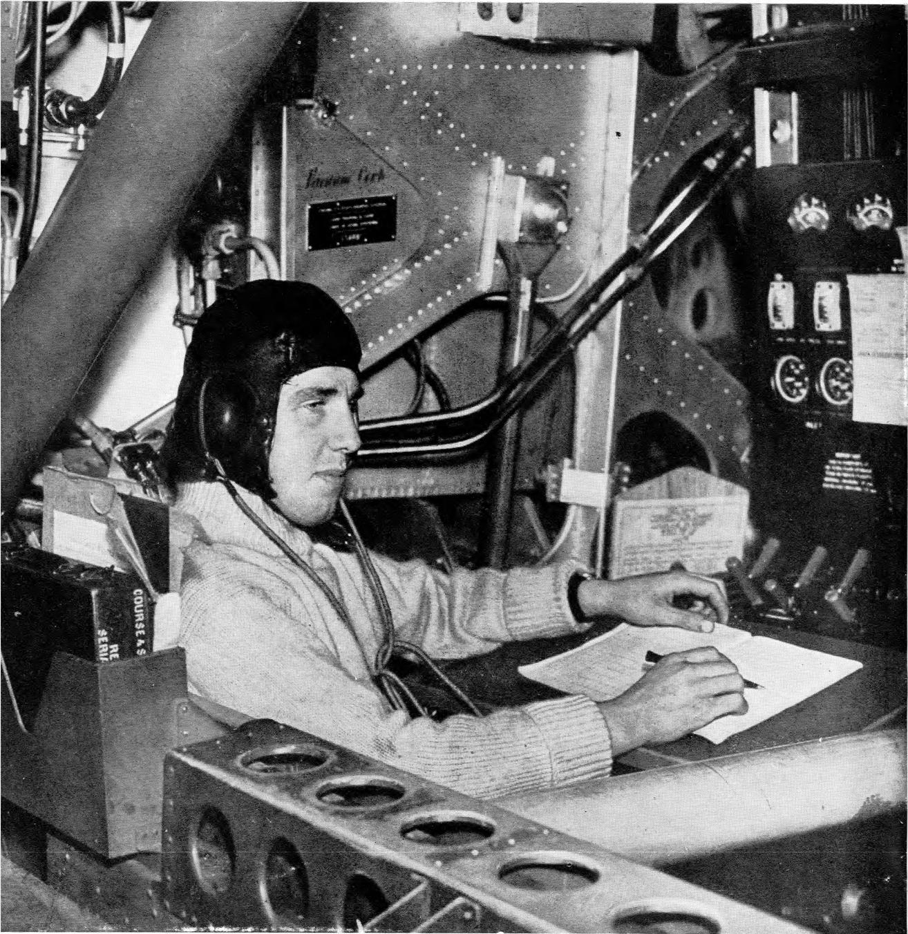
**The flight engineer** watches his instrument board, which tells him how the engines are behaving. Any fault must be corrected instantly, when an aircraft is so far from land.
