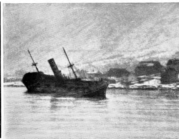
6. All resistance ceased in Narvik Harbour where the shore batteries were silenced and an enemy transport lay wrecked and aground.
