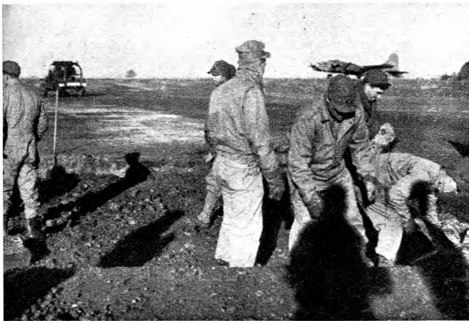
Repair: U. S. Engineers patch worn-out runways.
