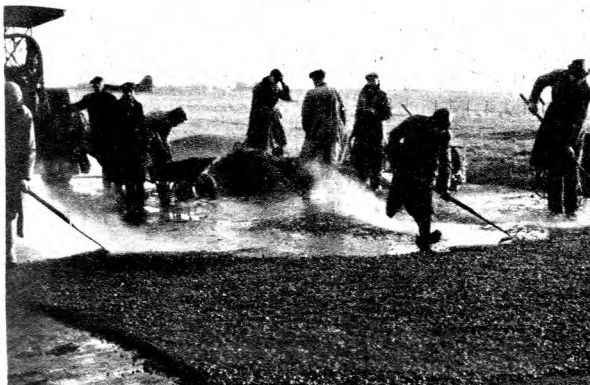
Construction: British labor works on a field for Forts.
