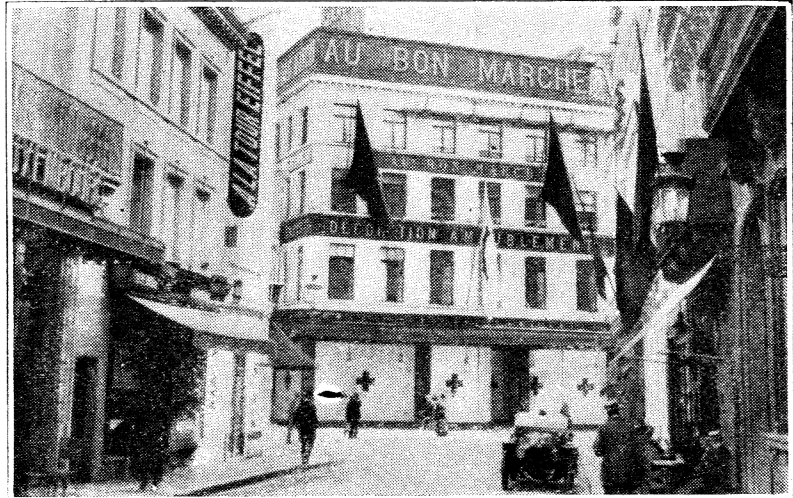
The Bon Marche shops as Red Cross hospital—windows marked.
